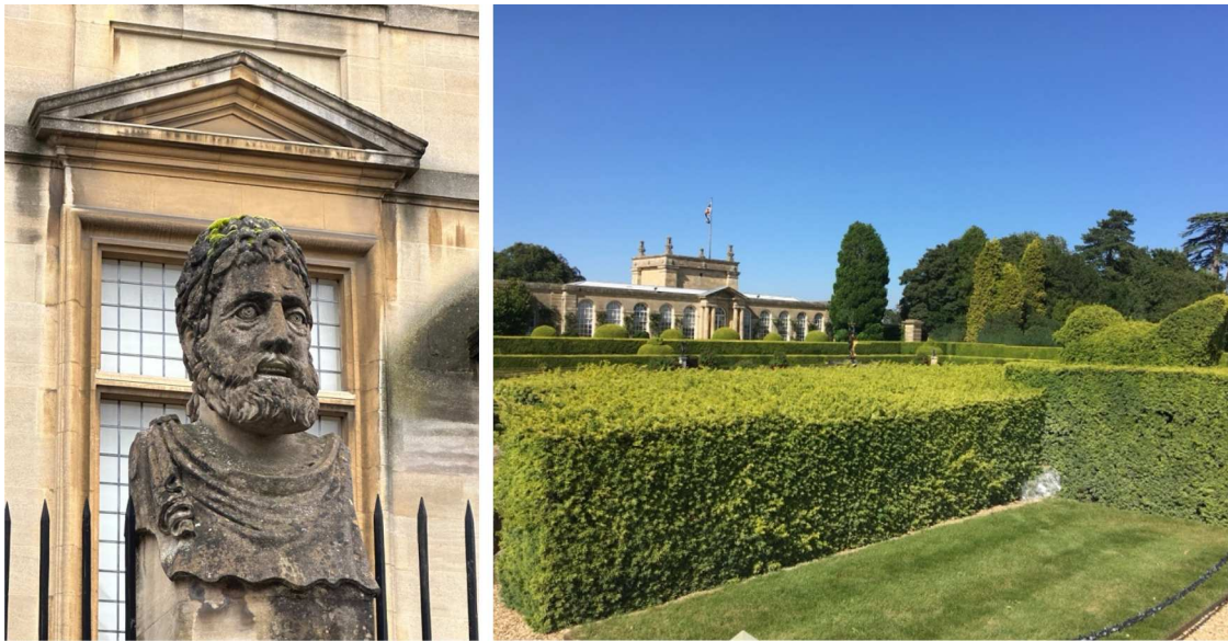
Figure 1. (a) One of the 'Emperors' Heads' from outside the Sheldonian Theatre, Oxford, UK. Carved from limestone by Michael Black in the 1970s to replace former, deteriorated sculptures, and subject to deterioration from climatic drivers and air pollution, with extensive cover of mosses and other organisms. (b) Formal gardens and parkland surrounding Blenheim Palace, Woodstock, UK which are part of the World Heritage Listing. (Images: author's own).
