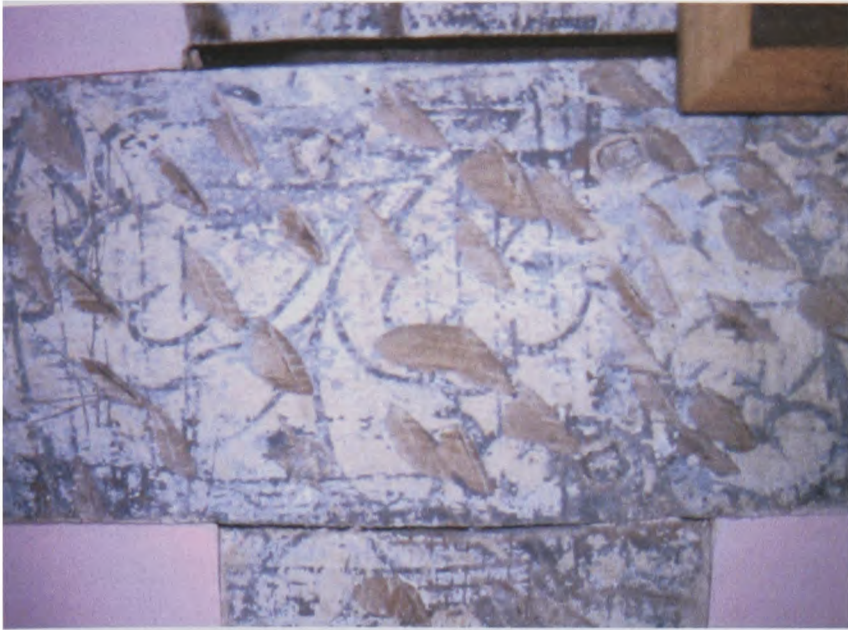
Fig.10.46 Crude panelling, Sutton Court Farm, Stanton, Shrops.
