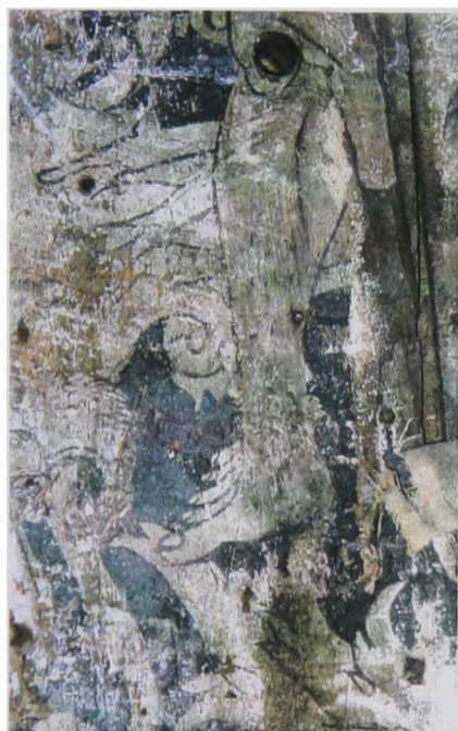
Fig.7.1 45, Muxton Lane, Telford, Shrops., showing linen covering joint
