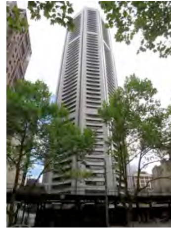
Figure 1.7: Nauru House, Melbourne
