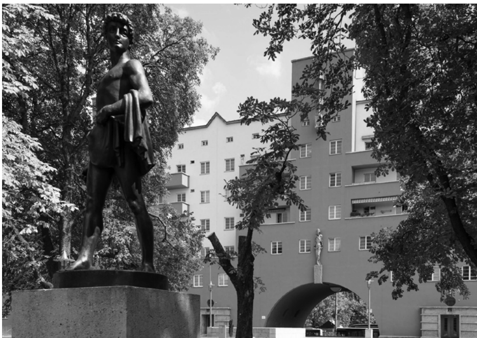
In The Great Transformation , Polanyi wrote that Red Vienna's attempt to transcend the market economy produced "one of the most spectacular cultural triumphs of Western history." Here, Karl-Marx-Hof, the longest single residential building in the world, completed in 1930. Photo by Jan de Boer.
