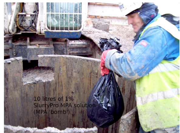
Figure 4.14: Dropping an MPA ‘bomb’ into a pile bore. (Photograph taken at the Castle House site in London.)
