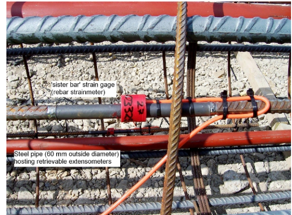
Figure 4.12: ‘Sister bar’ strain gauges and access tubes for cross-hole sonic logging and extensometer installation: left ) instrumented steel cage; right ) close-up.
