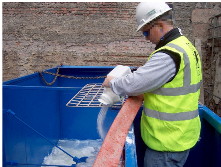
Figure 1.9: Sprinkling polymer granules into the mix water.
