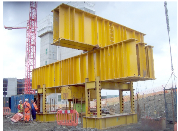
Figure 4.32: Reaction frame being constructed for the load test.
