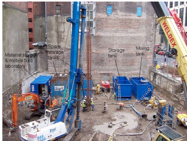
Figure 1.8: Photograph of a site in Glasgow where polymer fluids were used.
