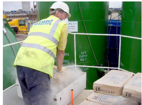
Figure 4.17: Adding bentonite powder into a mixer.
