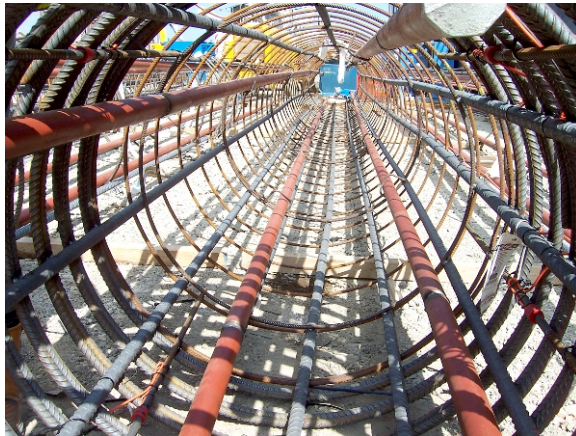
Figure 4.12: ‘Sister bar’ strain gauges and access tubes for cross-hole sonic logging and extensometer installation: left ) instrumented steel cage; right ) close-up.
