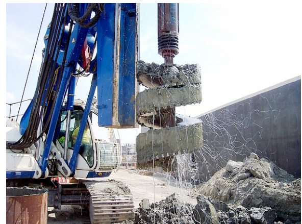
Figure 1.3: Piling auger immediately after extraction from a polymer-supported bore.
