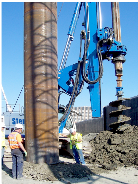
Figure 4.18: Temporary casing.
