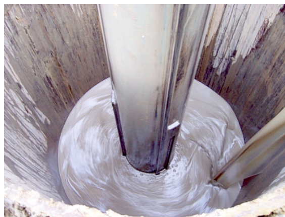
Figure 3.29: SlurryPro CDP polymer fluids after repeated use at the Castle House site.
