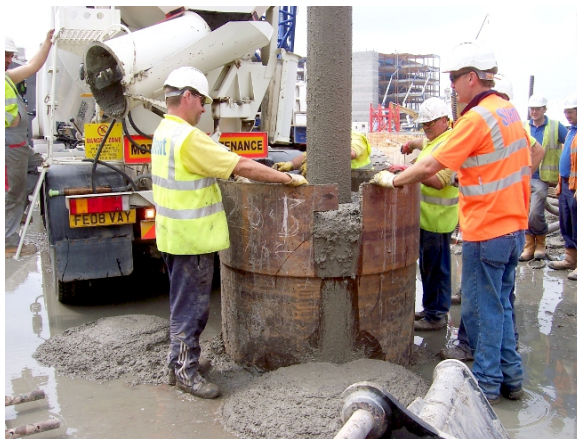
Figure 4.25: Tremie concreting.
