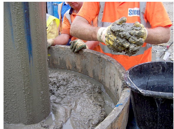
Figure 4.26: Taking samples from the concrete-support fluid interface.
