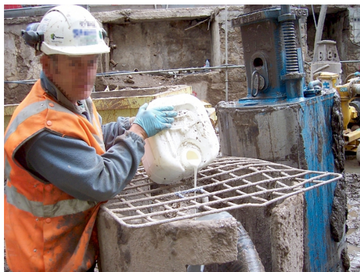
Figure 1.10: Adding emulsion polymer directly into a pile bore.
