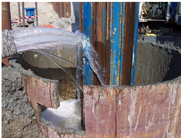
Figure 1.2: Polymer fluids being pumped into a pile bore.
