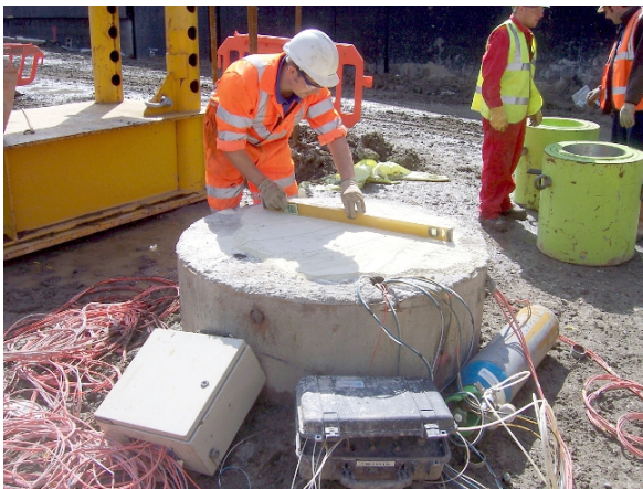
Figure 4.31: Preparing pile head for the load test and some instrumentation equipment on the ground surface.
