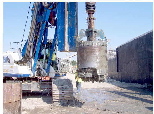
Figure 4.19: Vented digging bucket – note the teeth at the base.
