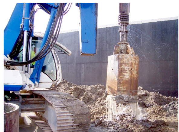
Figure 4.21: Flat-sided cleaning bucket – note the teeth at the base are replaced with a scraper plate.
