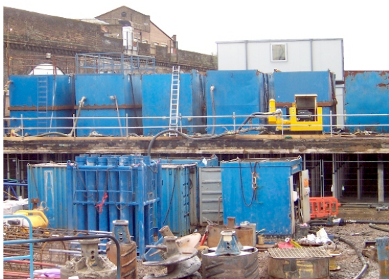
Figure 3.28: Photograph of tank layout at the Castle House site.
