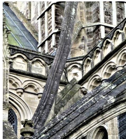
Fig. 7.6 Salisbury, north-east tower archebuttoon , J. Branche, 1481
