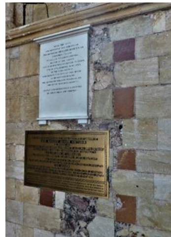
Fig. 8.6 Exeter, south nave aisle, scar of Norman respond repeated through south aisle
