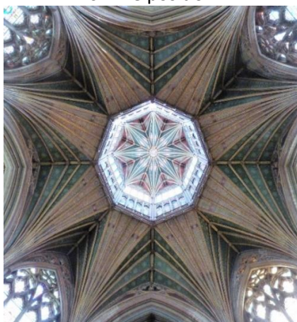
Fig.5.18 Ely Octagon timber dome and lantern vaults, William Hurley (1334-1342)
