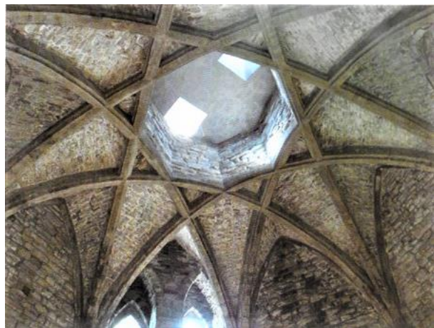
Fig 8.25 Durham, Prior’s Kitchen, 1366-74, John Lewyn, parallel ribs of the octagon vault
