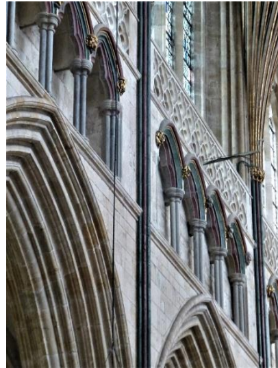
Fig. 7.17 Exeter presbytery, 3 stage with triforium inserted, 1317-18
