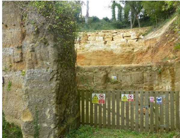
Fig. 10.2 Quarry, Dunscombe Manor, E. Devon, medieval face with pick marks to left, green and honey hues of Salcombe stone.
