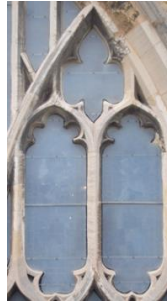
Fig. 9.1 Exeter Cathedral, great east window, lights A2-3, cusped stonework by Robert Lesingham, 1390, before recent restoration. Courtesy J. Allan
