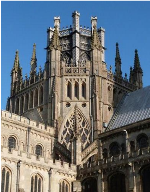
Fig 8.14 Ely Octagon, north-west, stonework, 1322-1326, attributed to John Ramsey; timber lantern above
