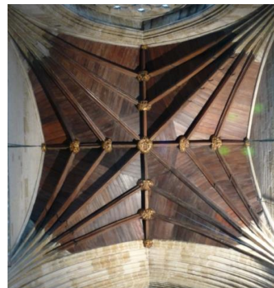
Fig. 9.7 Exeter Cathedral, north tower/transept timber vault, nine bosses, Witney (1317-18)
