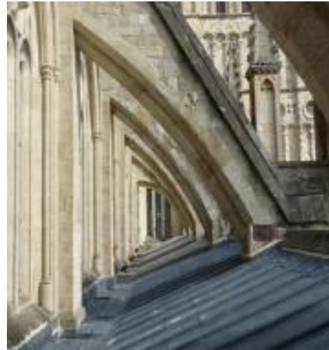
Fig. 9.9 Exeter Cathedral, south aisle inward sloping roof, Thomas of Witney, 1331-32.
