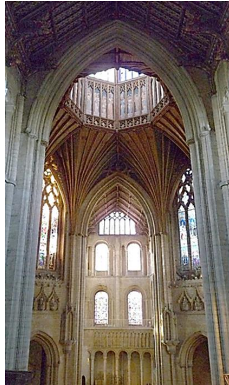
Fig 8.15 Ely Octagon, vaulted dome and lantern, 1327-1342, after William Hurley
