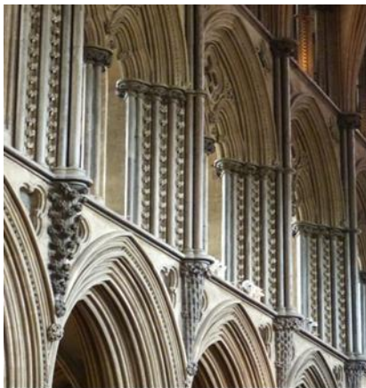
Fig. 5.16 Ely, Northwold's Presbytery (1233-1250), bays 4-5 gallery showing unfurling stiff-leaf corbels at base of vaulting shafts, indicating shrine position
