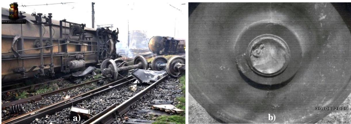
Figure 1. Images from the Viareggio train derailment (Italy). a) Capsized carriages and detached wheel sets [2]. b) Detail of the axle failure due to fatigue [3]
