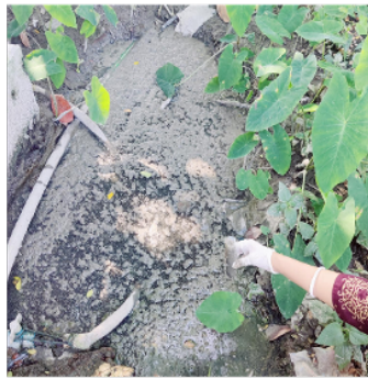
Drain near the hospital
