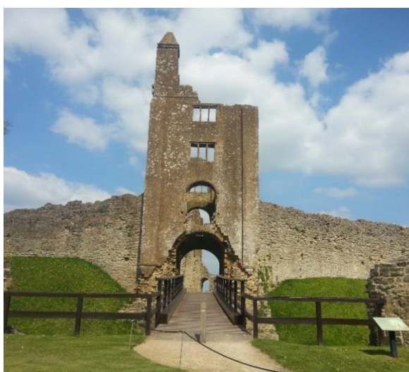
Figure 5a: Sherborne gatehouse, upper level (above top window) later addition 95
