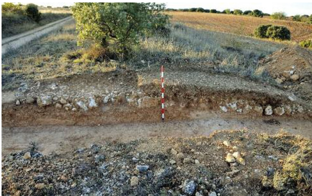
Figure 2: Photography of the Via from Clunia to Segisamo (Castille and León), where the foundation of large limestone rocks and a surface layer of natural ballast over it can be appreciated. Source: Moreno, (2004:24) (used with copyright-holder's permission).
