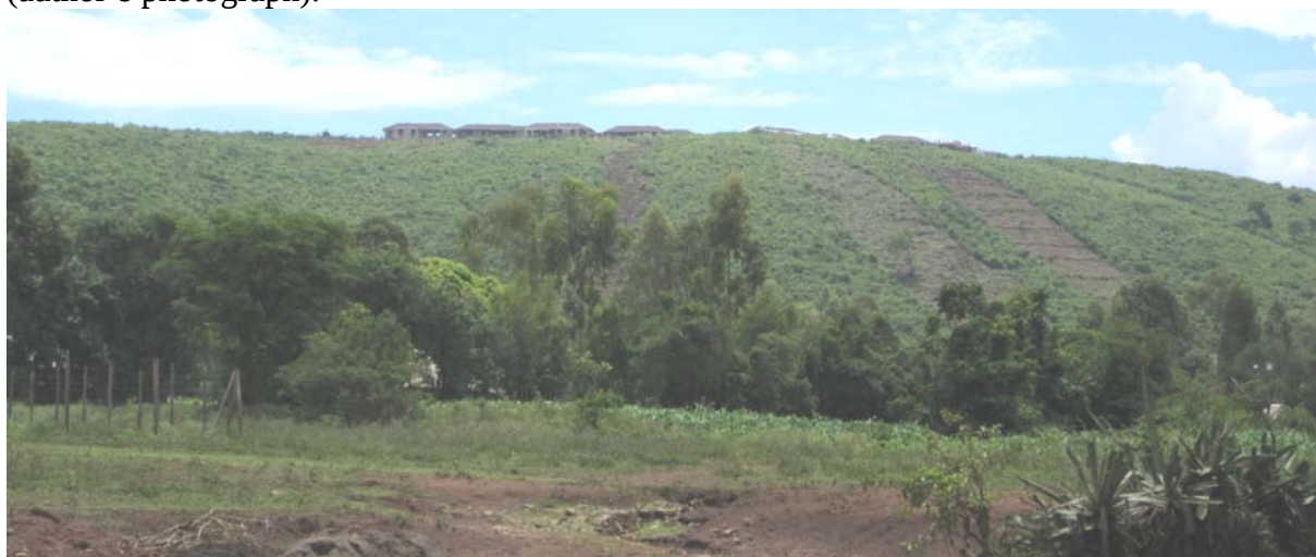
Fig. 7.2: The new SOS Children’s Village, situated above the existing village (author’s photograph).
