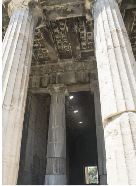
Fig. 10. View of the barrel vault in the Hephaestion in Athens. During the later medieval reconstruction of the building, holes were added in the new vault, possibly to improve illumination or air circulation. Courtesy of ancient-greece.org.
