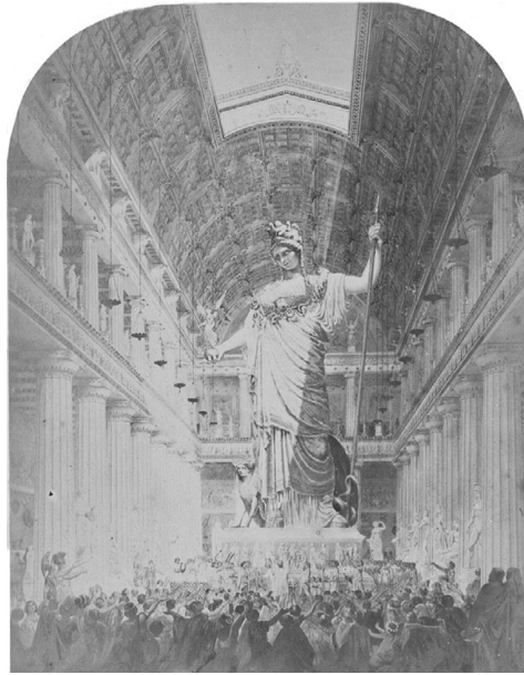
Fig. 2. View of the interior of the cella of the Parthenon, following Quatremère de Quincy models, by Edward Falkener (British, 1814–96). J. Paul Getty Museum, Los Angeles, 84. XB.944.4.1. Photo: Falkener 1861.
