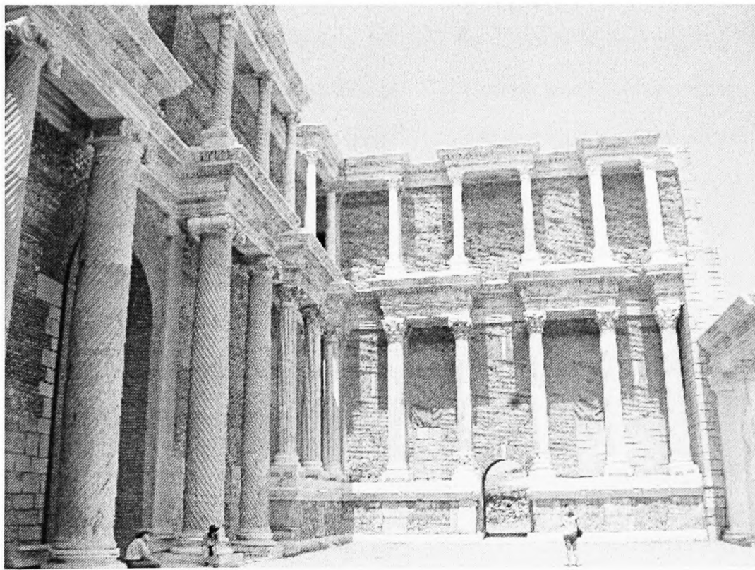
Figure 20 Kaisersaal in the bath-house at Sardis. Photograph: author.
