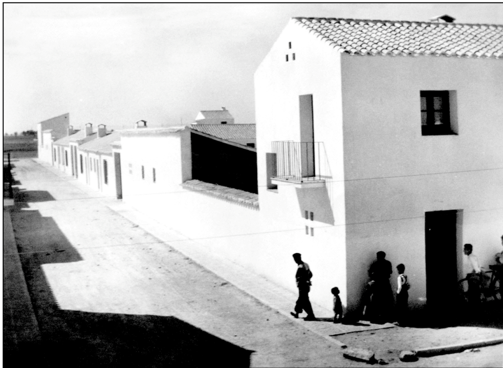
Photograph 5.7 Street view in Llanos del Caudillo, 1950s
