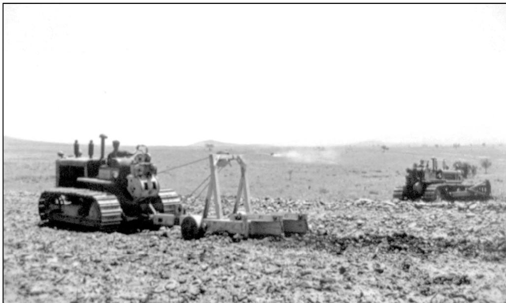
Photograph 5.2 Ground levelling by the INC in La Mancha, 1950s
