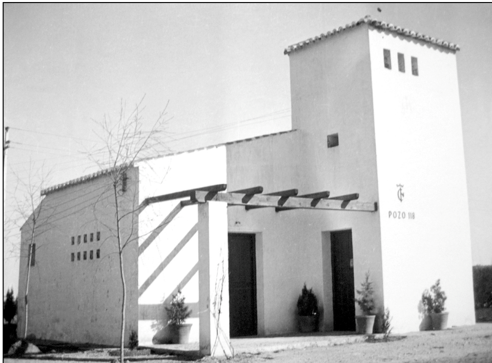
Photograph 5.4 Electric transformation station for a well in Llanos del Caudillo
