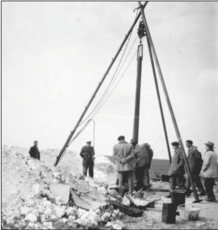
Photograph 5.4 Drilling with percussion technology in Llanos del Caudillo, 1950s
