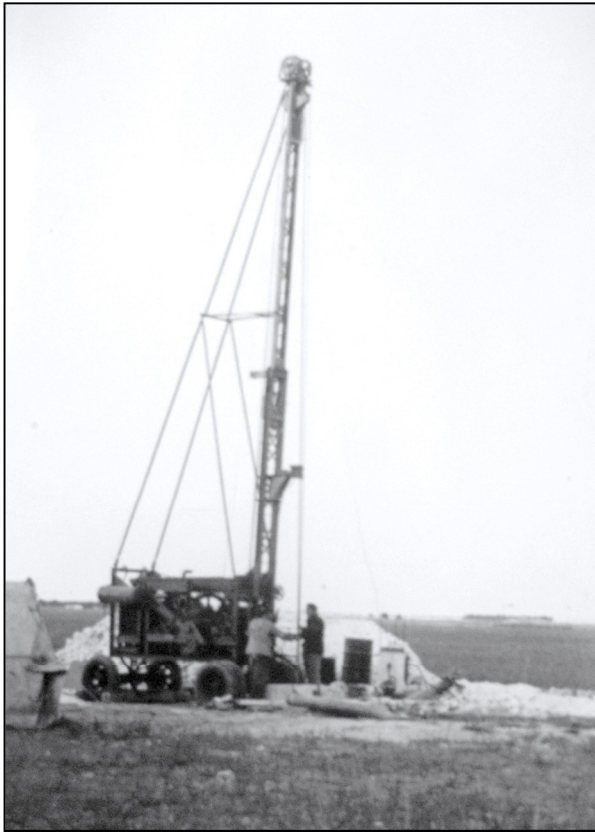
Photograph 6.5 Drilling equipment in La Mancha, 1950s
