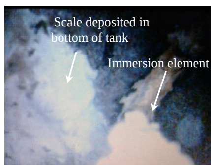
Figure 3-8 Image of bottom of tank taken from endoscope
