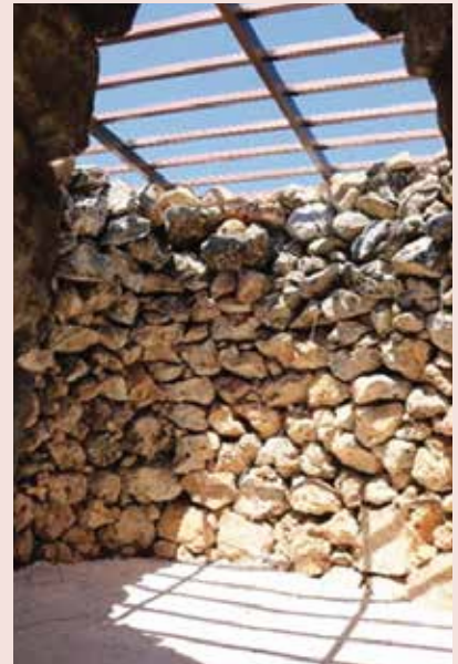
Using traditional materials and techniques during the conservation of watchtowers at Al- Makhrou area (Photos by Ziad Abuowda)
