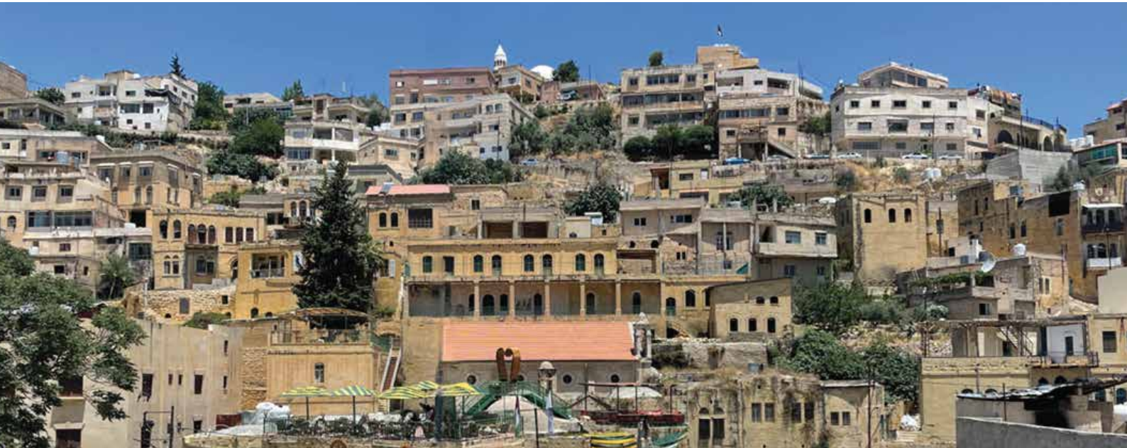
Figure 10 General view of As Salt World Heritage Site. Photo by H. Abedalhaleem
