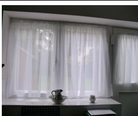
Figure 219: TSB034, kitchen window above the sink problem in operation due to the width of wall insulation, height of the handle position and reaching distance from the user.
