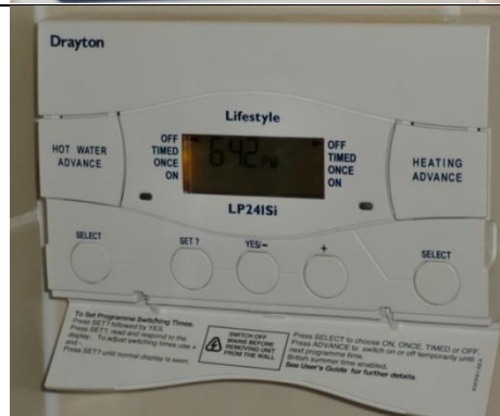
Figure 192: Convectional programmer.
