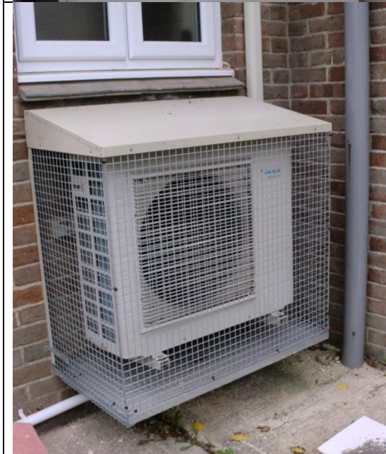
Figure 147: Air to air source heat pump (Daikin), TSB097.
