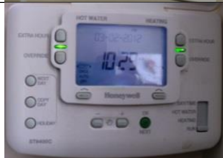
Figure 193: Convectional programmer.
