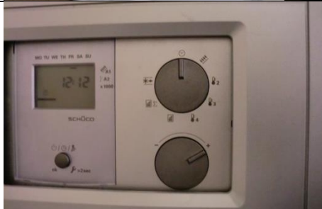
Figure 206: Solar thermal controls.
