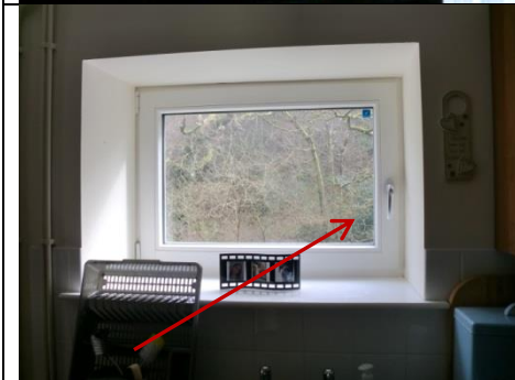
Figure 224: TSB069, kitchen window above the sink problem in operation due to increased insulation thickness of the wall and reaching distance for the user.
