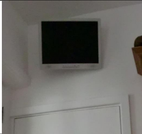
Figure 187: Monitoring display real time energy display monitoring energy consumption for the 'whole house' and individual appliances.
