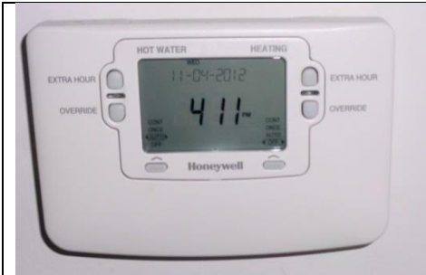
Figure 195: Convectional programmer.
