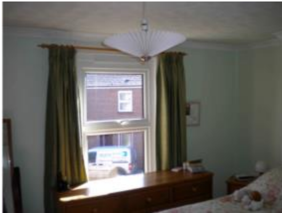
Figure 48: Base case double glazed window, tilt opening type with trickle vent.
