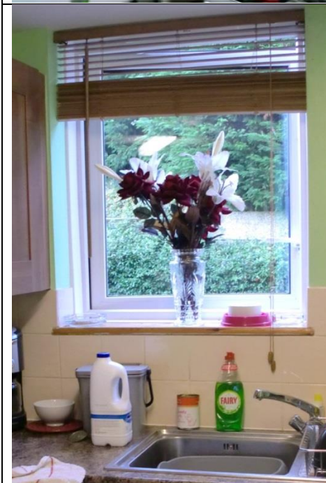
Figure 227: TSB076, kitchen window above the sink problem in operation to be fully opened due to the handle's reaching distance from the user.
