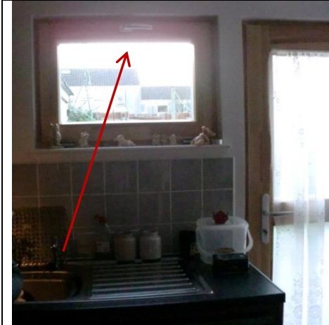
Figure 223: TSB042, kitchen window above the sink problem in operation due to the height of the handle position and reaching distance from the user.
