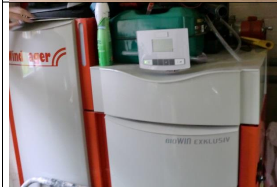
Figure 145: Domestic biomass boiler (TSB002).
