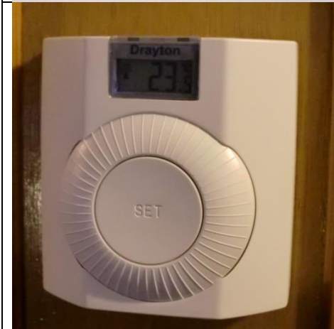
Figure 197: Digital thermostat.
