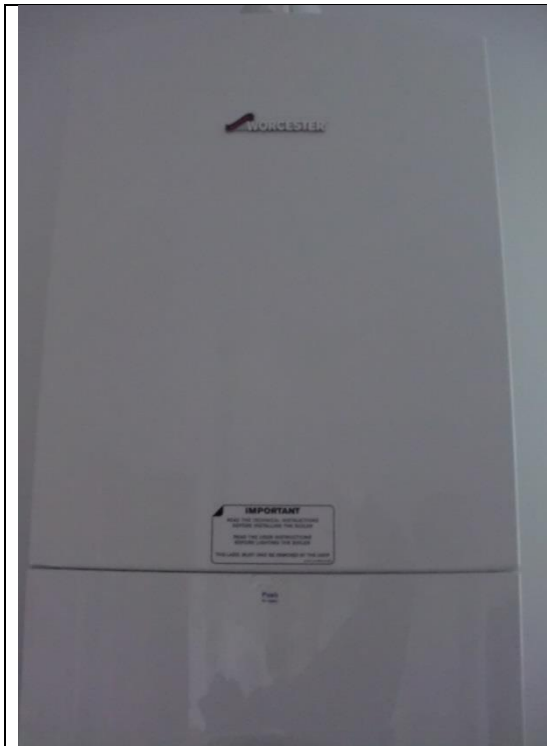
Figure 150: Combi gas oiler (Worcester Greenstar 25Si) (TSB113 and 098).
