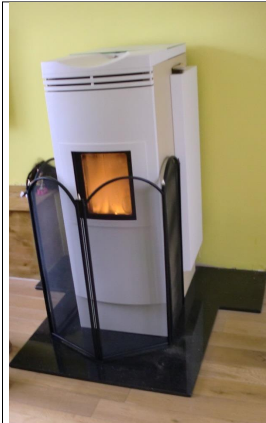
Figure 144: Domestic biomass boiler (indoor living room) (TSB087).
