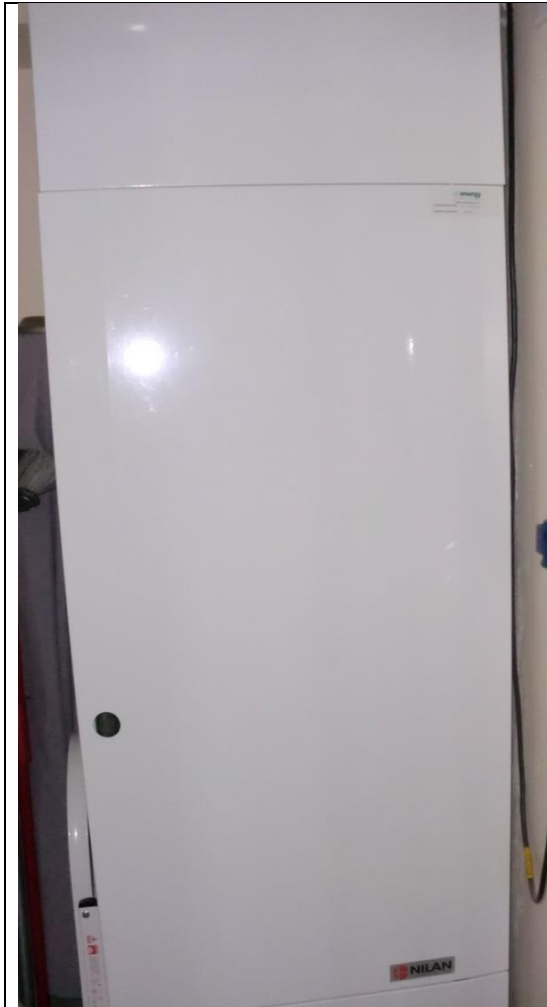
Figure 146: Air source heat pump ( Nilan VP18 compact heat pump ASHP for Ventilation with heat recover, space heating and domestic hot water production ), TSB031.
