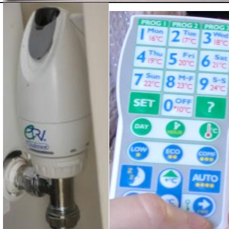
Figure 190: Intelligent TRVs (thermostatic radiator valves) with control settings.
