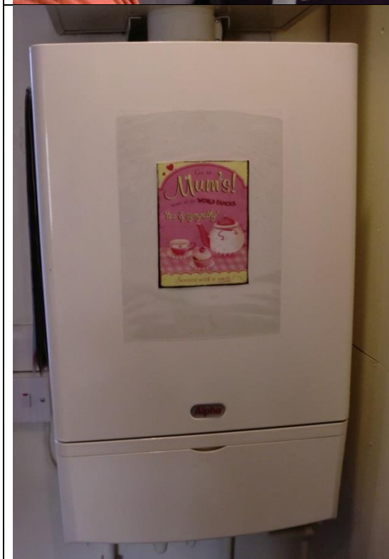
Figure 149: Condensing gas boiler (Alpha CD12S) (TSB027).
