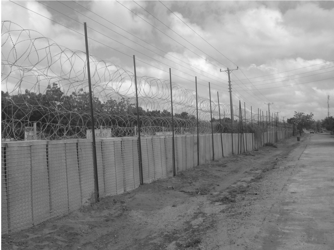
Figure 15: Perimeter fence at Dadaab Main Office, Dadaab (source: author 2017).
