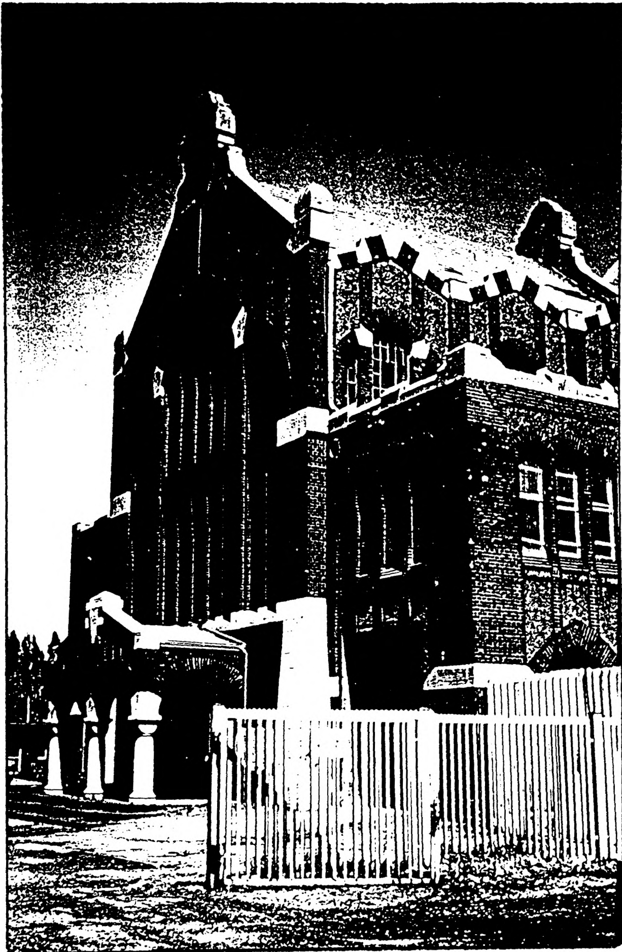
'Zeche Westhausen', pit-head building, Dortmund-Bodelschwingh 1904-5. Present condition.
