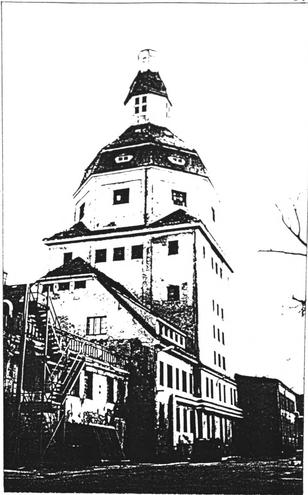
fig.42 Municipal abattoir - Power station, Dresden 1906-10. Arch. H.Erlwein. Present condition.
