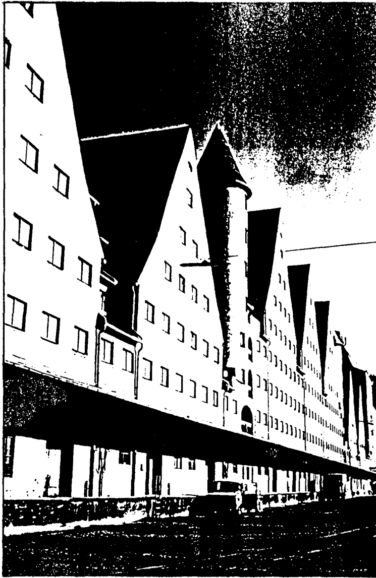
Municipal warehouses, Cologne-Agrippinaufer 1908-9. Arch. H.Verbeek. Present condition.
