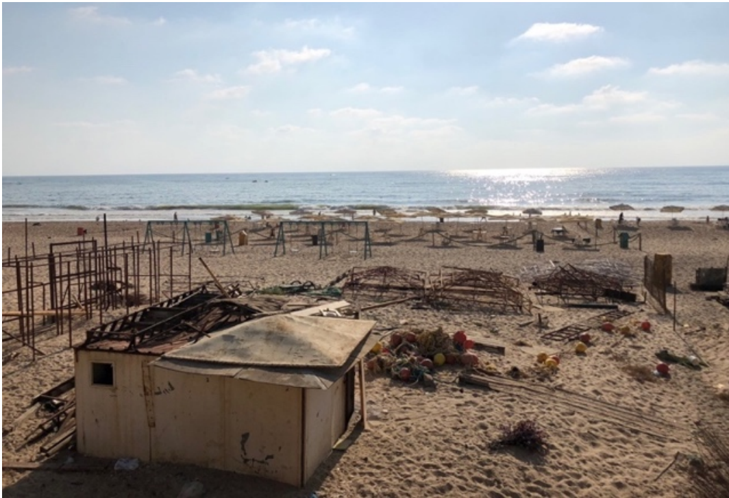
Figure 7. Dilapidated structures, Ramlet El Bayda. Source: Tarek Kheireddine
