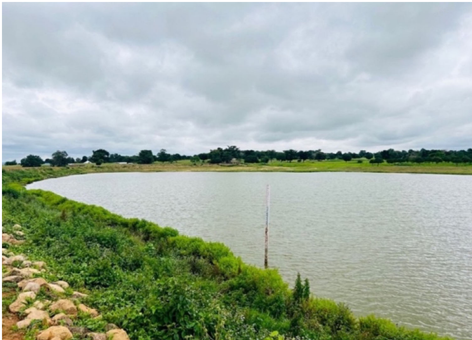
Figure 3: The rehabilitated dam in Bongo-Dua, Bongo (source: image captured by the author during fieldwork in Bongo)
