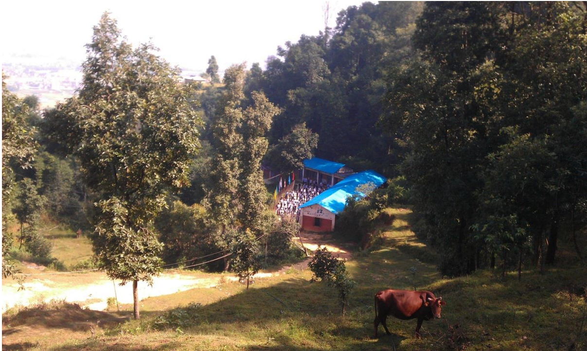
Figure 6 Aerial view of Bhumi
