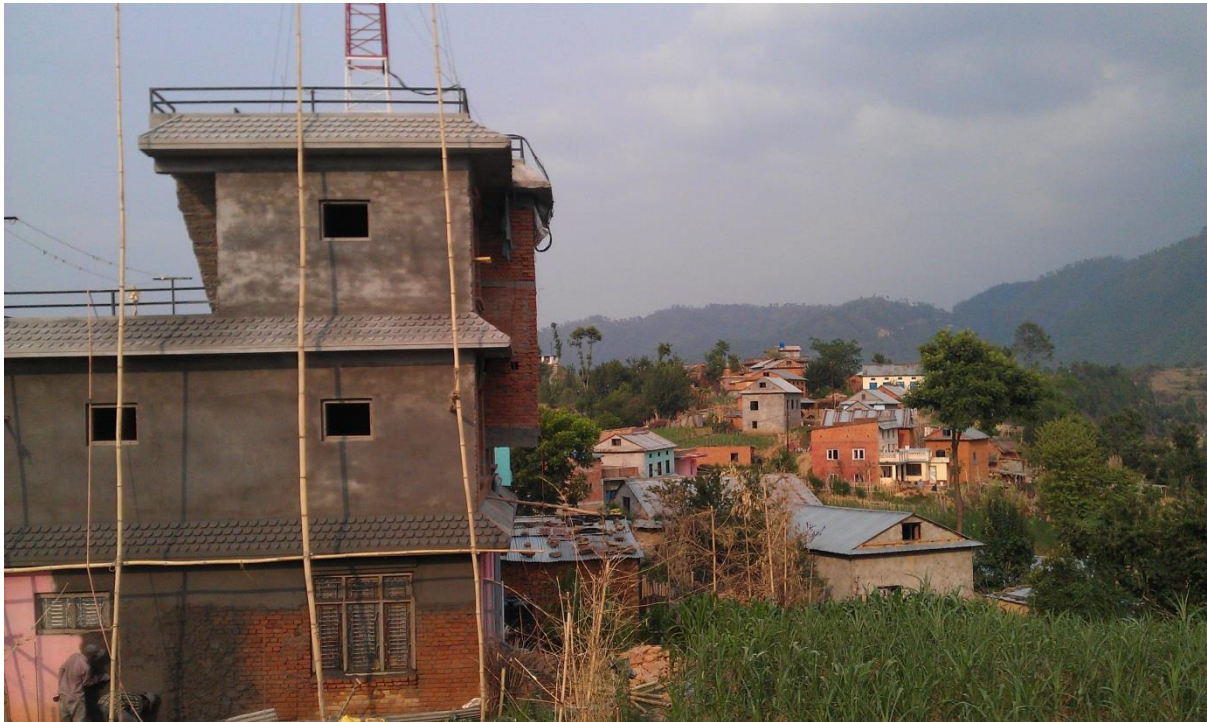
Figure 13 New construction in Dadagaun
