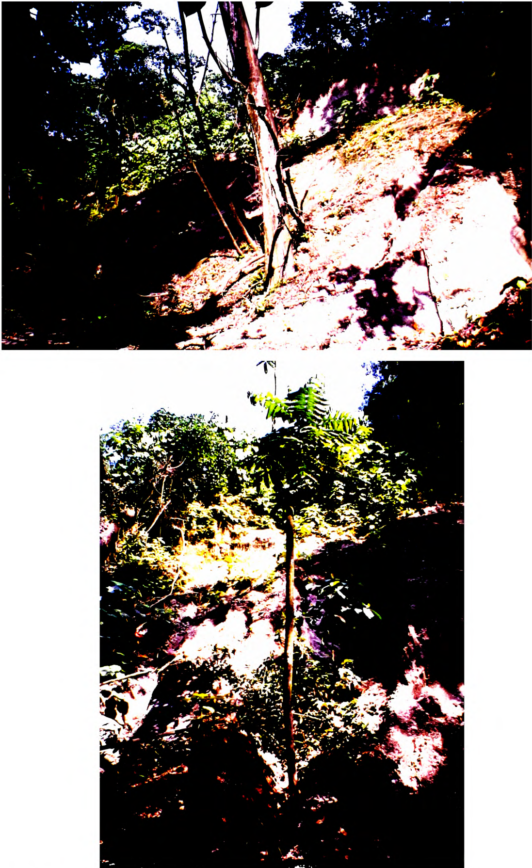
Fig. 2.12: Examples of pumice digging damage in near-coastal gullies of North-east Panjang.
