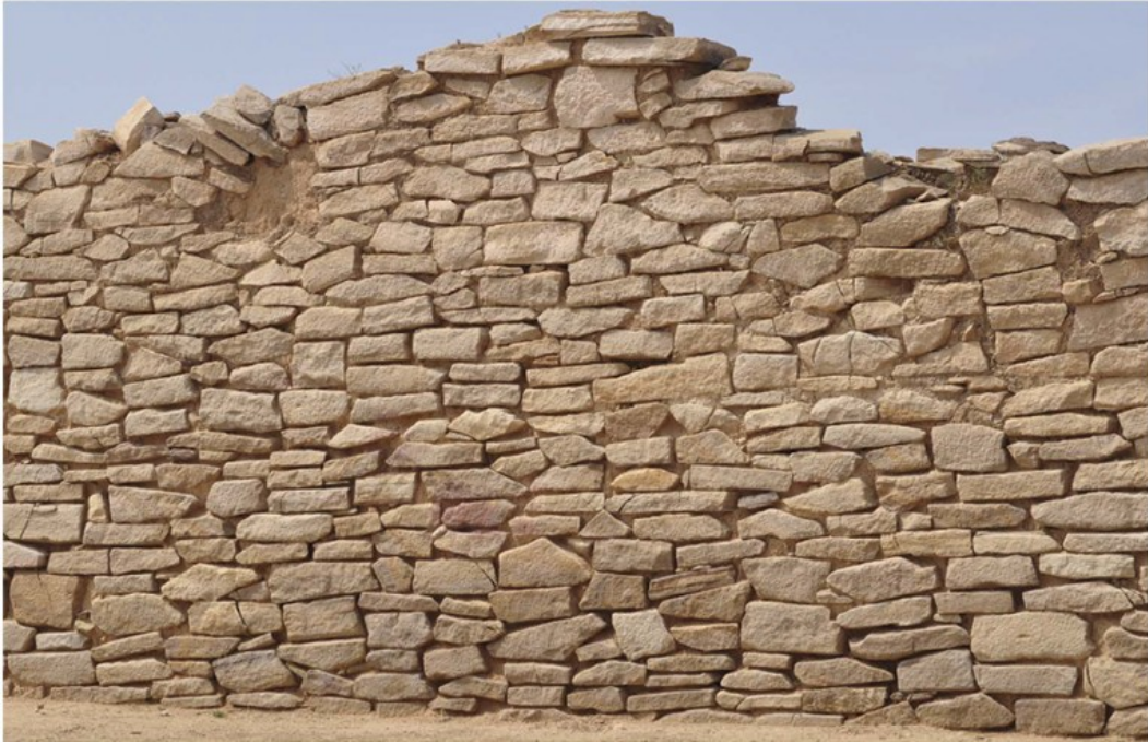
Figure 2.20. Photo of the wall construction at Huangchengtai, Shimao that shows the worked and carefully placed stone blocks. Figure from Jaang et al. (2018: 1018).
