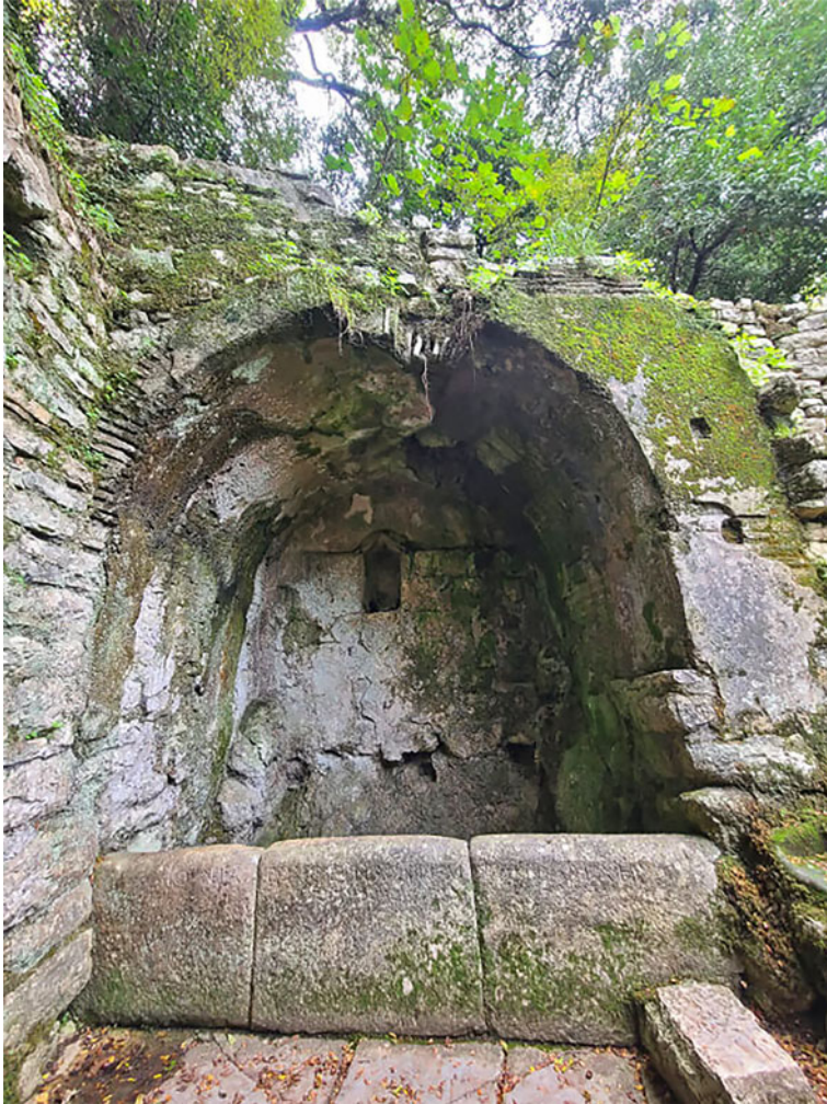
Fig. 4. Present condition of the well. (M. Melfi.)
