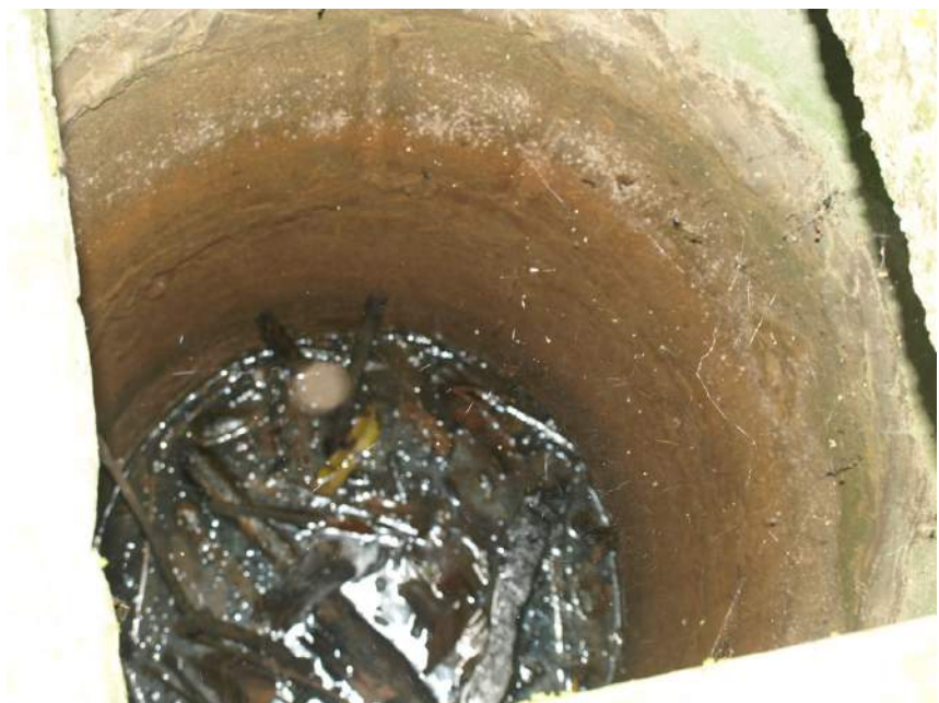
Figure 8. Looking down into a non-functioning well that was built by COTCO as reimbursement when a borehole was destroyed during pipeline construction, Mpango (Amber Murrey)
