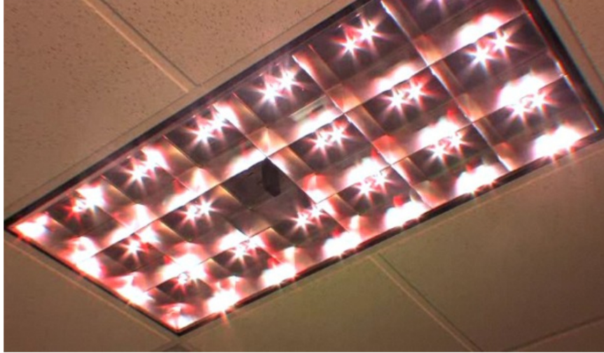
Figure 5. An example of an array of LED sources that is potentially used in VLC systems to provide sufficient illumination for an indoor work environment [67]. This array of LEDs provides independent channels, which can be utilised in MIMO transmission paths.
