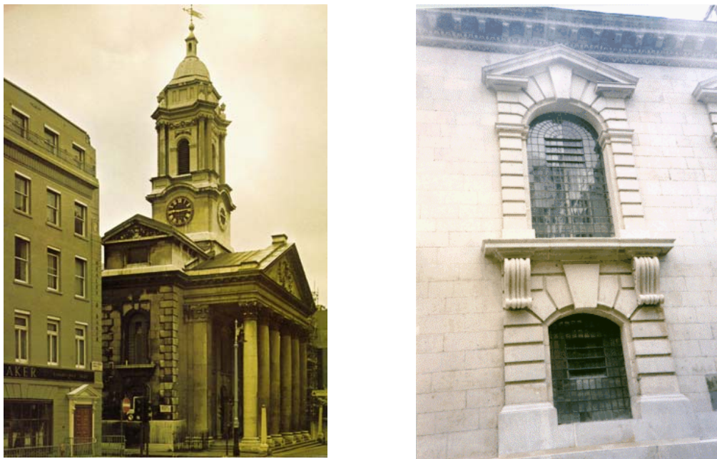
Figure 5-3: View to front of St George's Church and detail at arched window openings
