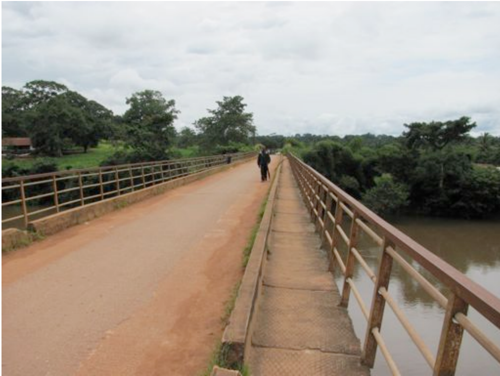
Figure 5: Daru Bridge, Kailahun District (2010).
