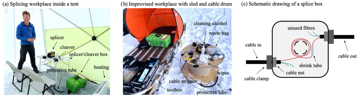
Figure 4. Optical fibre splicing in practice. (a) Splicing workplace set up in a tent near the EastGRIP camp site on the Northeast Greenland Ice Stream. Ideally, splicing should be done by a team of two in an environment that allows for focused work for potentially several hours. (b) An improvised workplace setup on a sled and a cable drum at several kilometres distance from the EastGRIP camp. (c) Schematic drawing of a splice box. An important feature that not all commercially available boxes have are the cable clamps that offer some tensile strength, which is important in the field.
