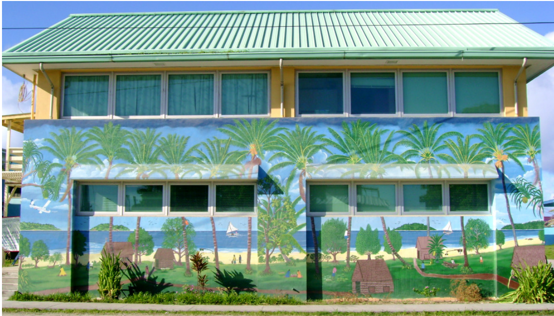
Figure 1. Mural on the exterior of the Youth to Youth in Health building, Majuro
