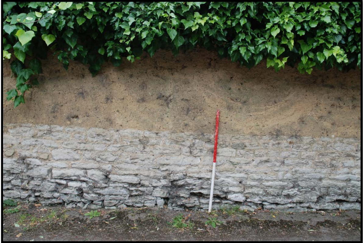
Figure 5. 8: Cob wall, based on Upper Greensand footing, at the Fleur de Lys pub, Dorchester on Thames.
