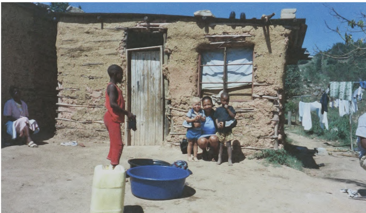
Figure 2: a home in an informal settlement within the Mbabane Municipal Boundary
