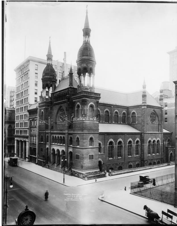
Figure 83. Temple Emanu-El, corner of West 43rd Street and Fifth Avenue, by Henry Fernbach, 1868. (Museum of the City of New York)
