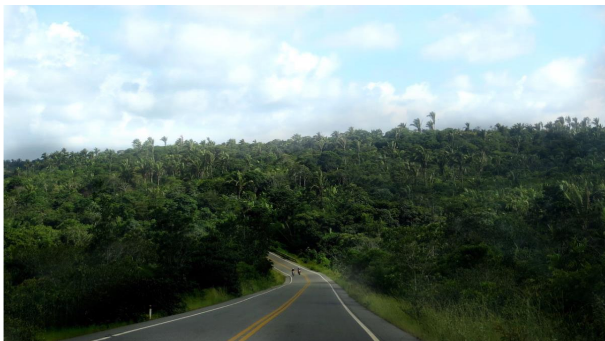
Picture 16: View of the MA-106 that connects Alcântara with the port and towns in the Baixada Maranhense.
