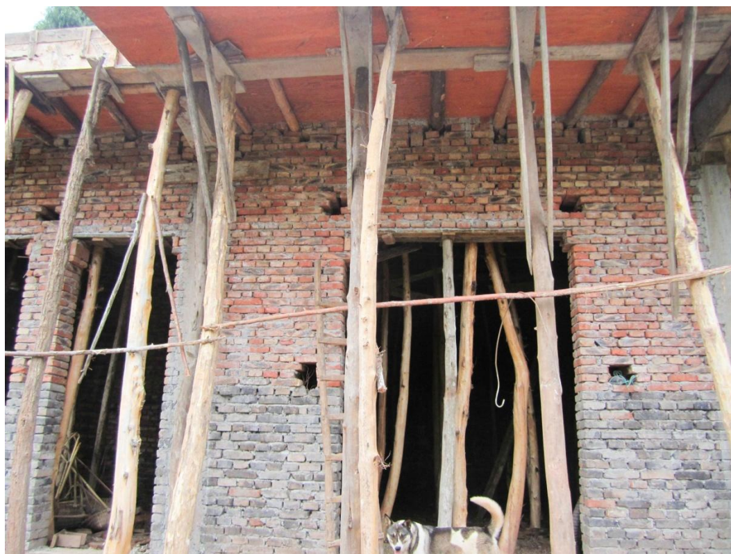
Figure 45. The Li's family house under construction.
