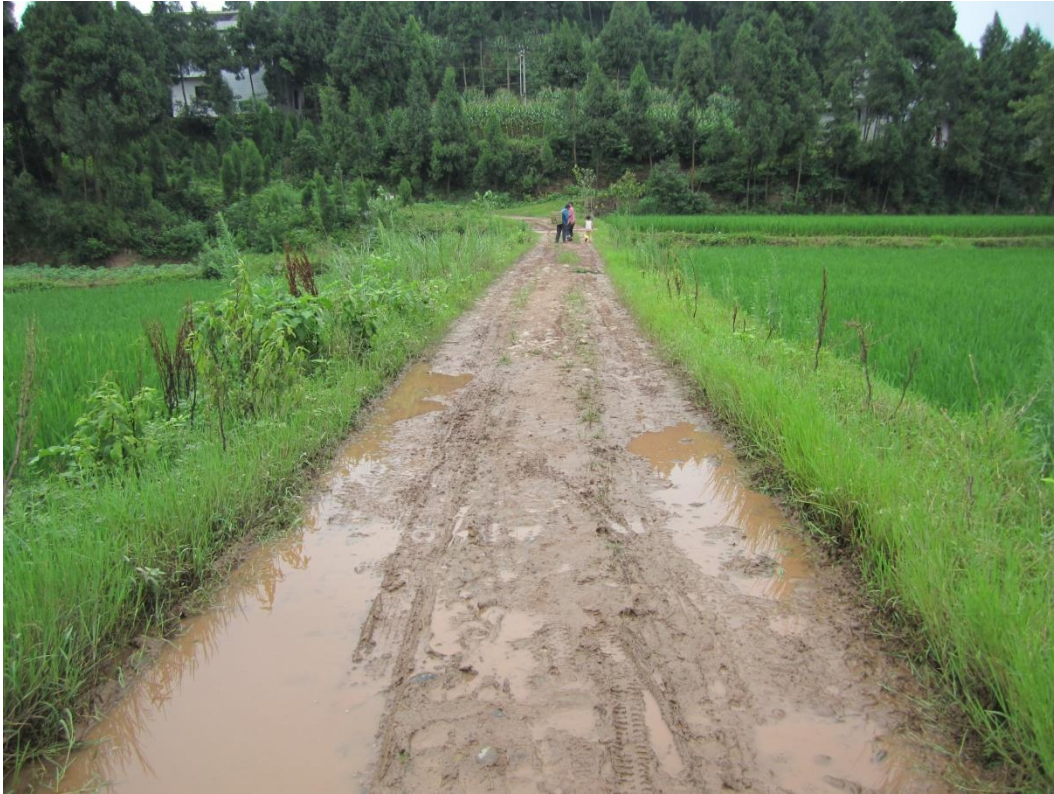
Figure 22. Unpaved road in Meijia.
