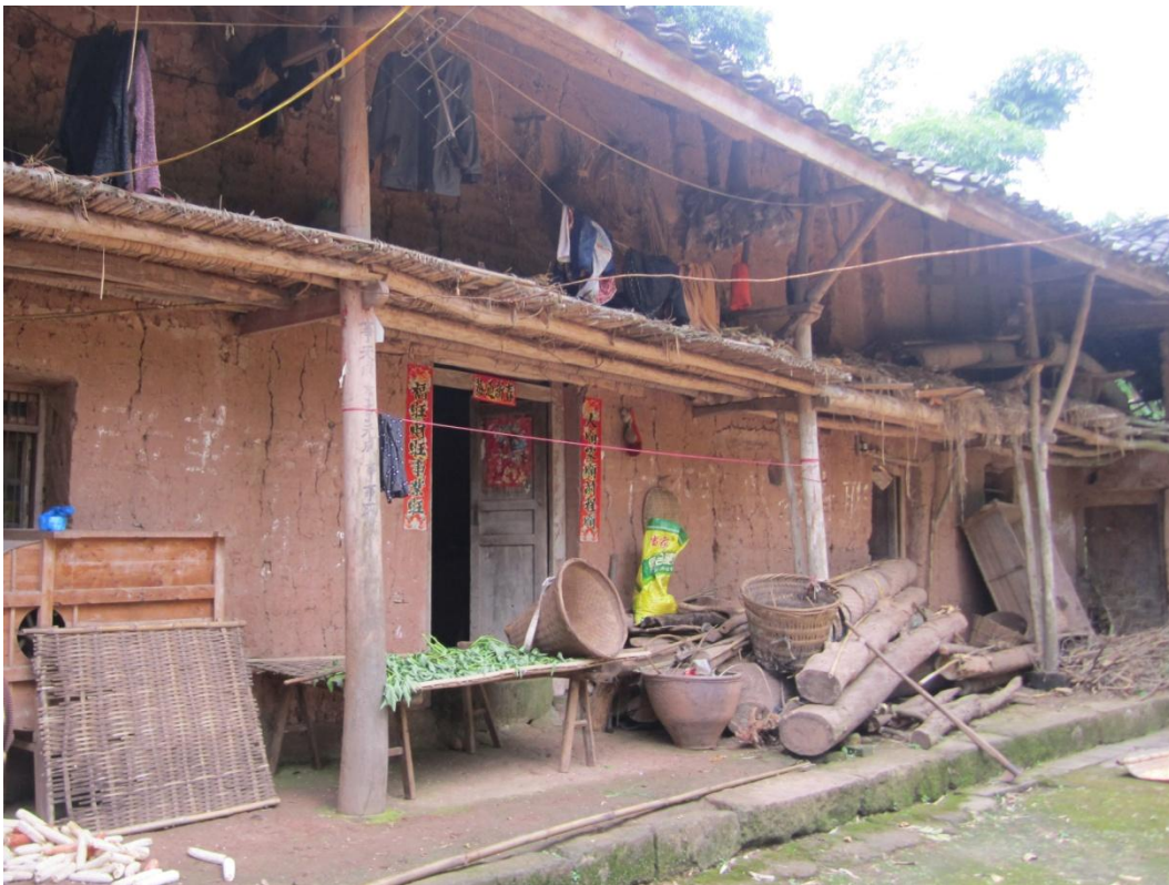
Figure 27. The Cai family has not built a new house.
