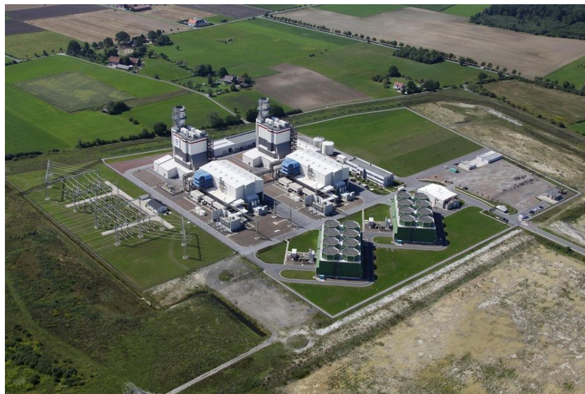
Figure 5: 850 MW CCGT at Hamm Uentrop, Germany
