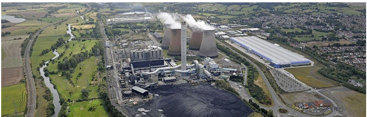
Figure 7: 1,000 MW Coal-Fired Plant, Rugeley, UK
