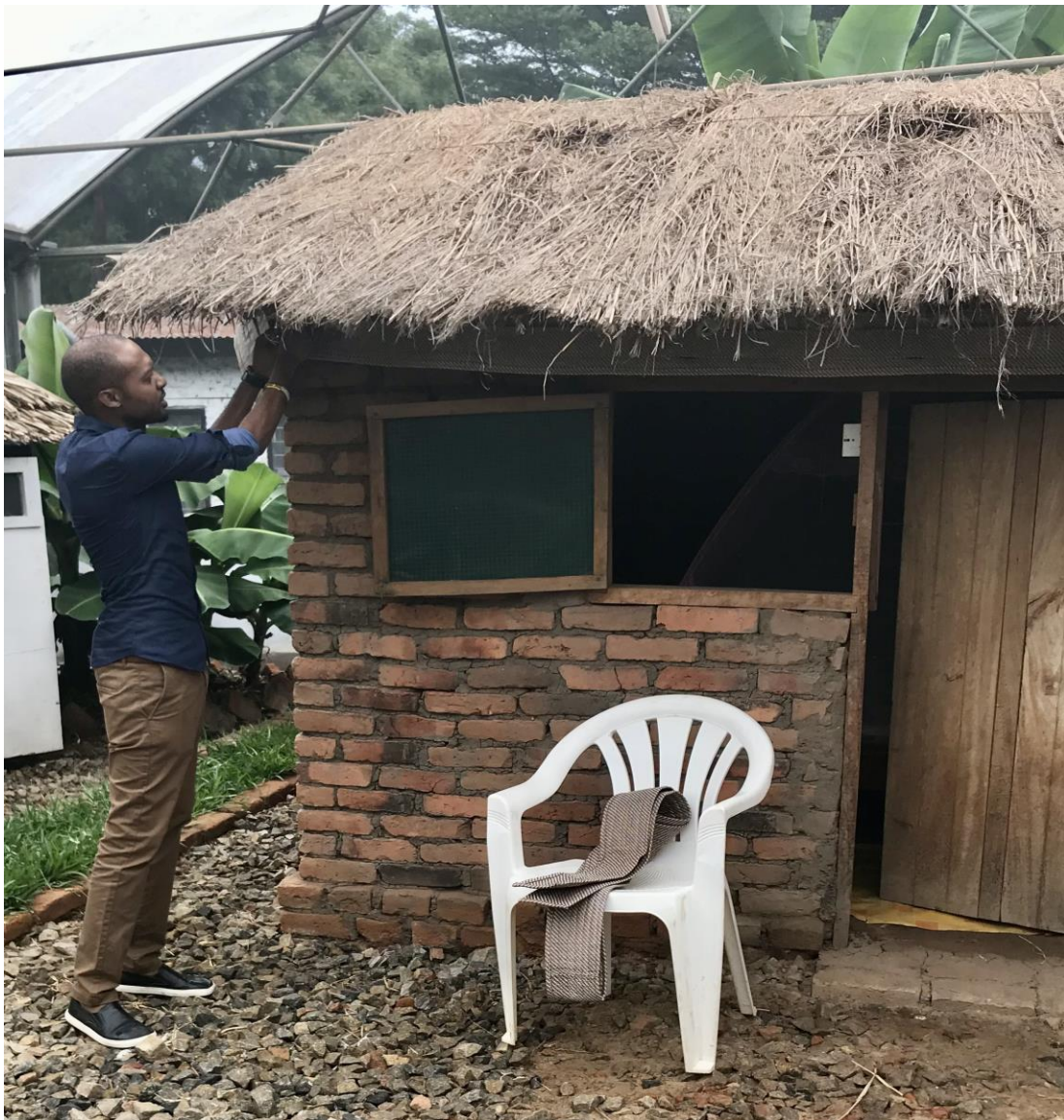
Figure 1: Arnold Mmbando affixing eave ribbons to an experimental hut, Ifakara Health Institute. Photo by the authors.
