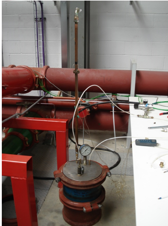
Figure 7.7. Flow calibration and pressure testing rig.
