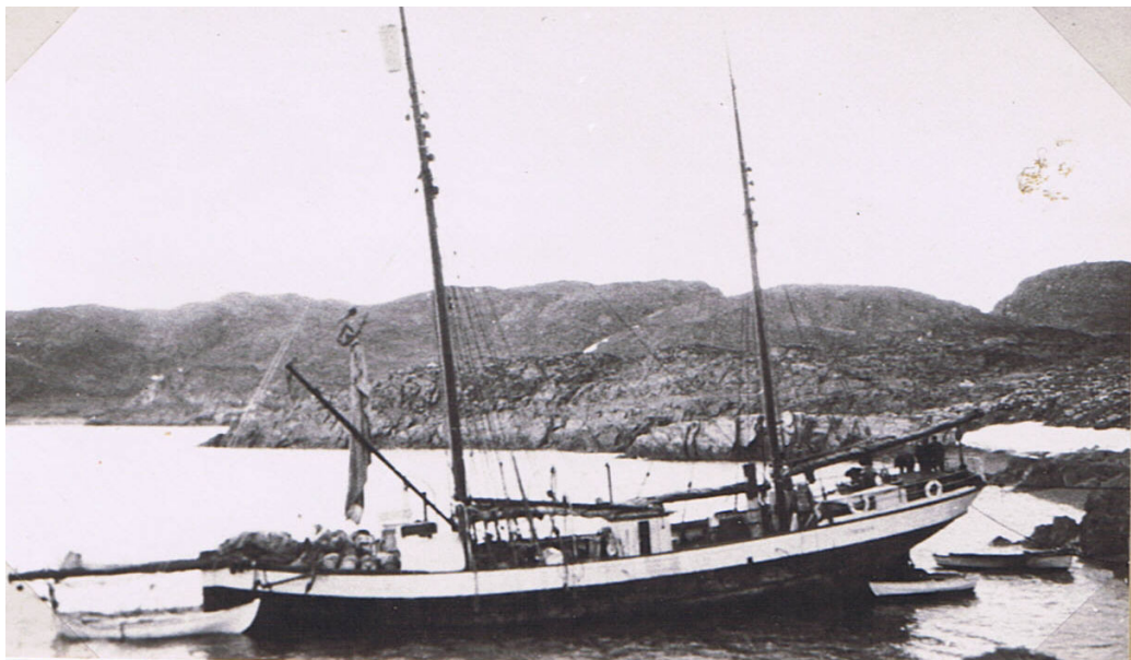
"Terningen" beached (a 4½ ft. tide) in Wijde Bay, to have propeller changed. Note whale-boat full of water weighing down bows, and goods piled forrard. 16 August 1923. (Photo T.G. Longstaff).
