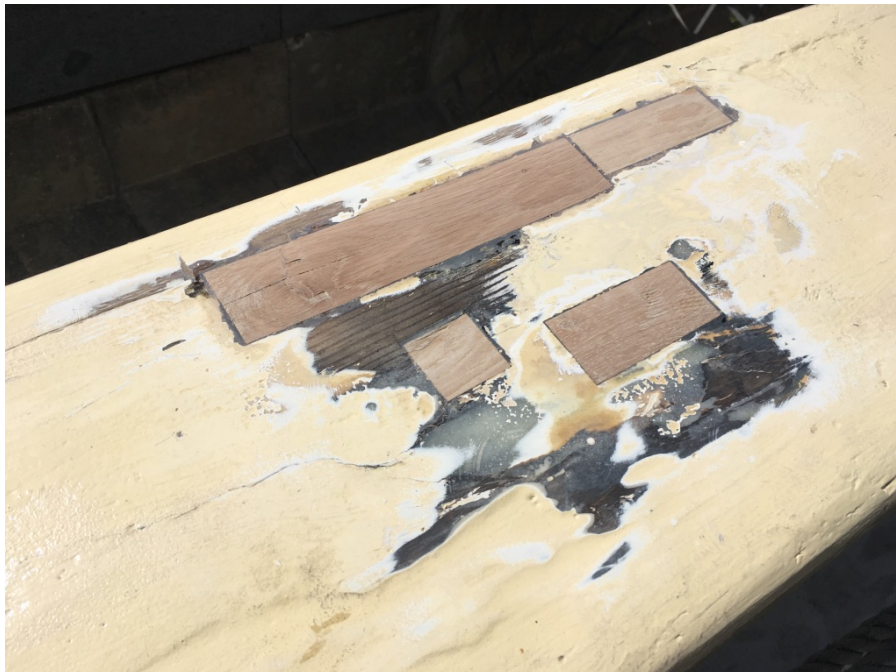
Figure 18: Dutchmen that I installed in the rail
