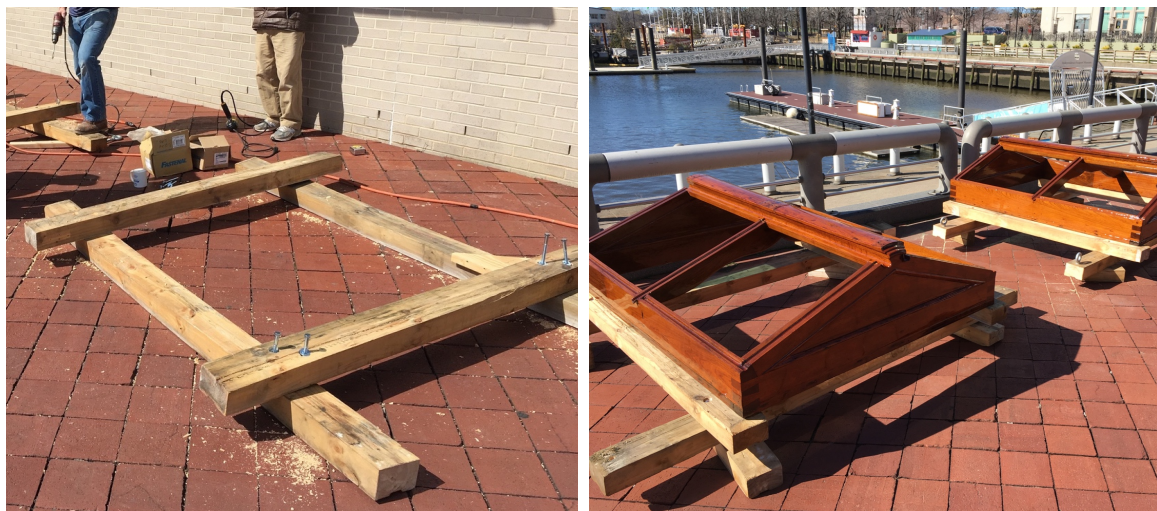
Figure 26: The cradles under construction (left), and the cradles in use (right)
