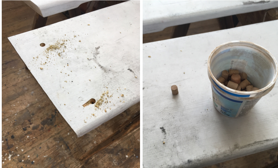
Figure 32: Bung-holes to be filled (left); a cup of newly-fashioned bungs (right)
