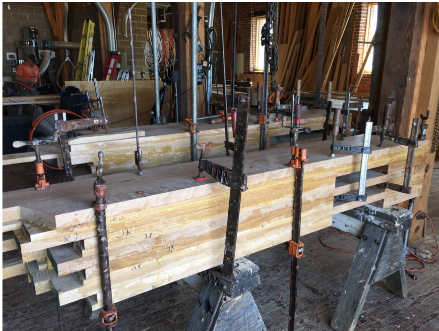
Figure 40: The new cat-heads under construction
