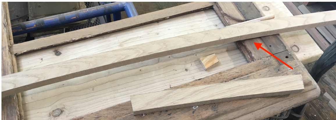
Figure 37: One of the deck beams before being installed
