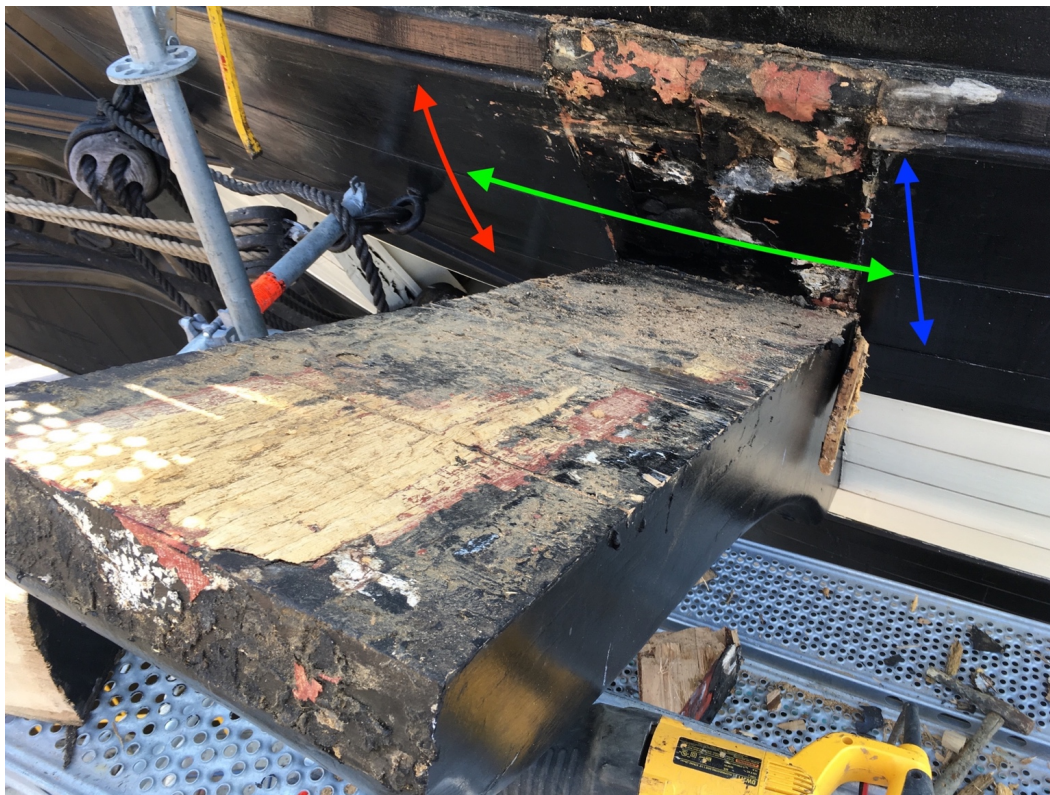
Figure 42: The hull of the ship where the cat-head will meet it. The wooden platform in the foreground is the 'knee'.
