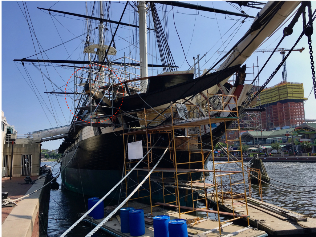
Figure 12: The starboard cat-head, partially demolished (circled)
