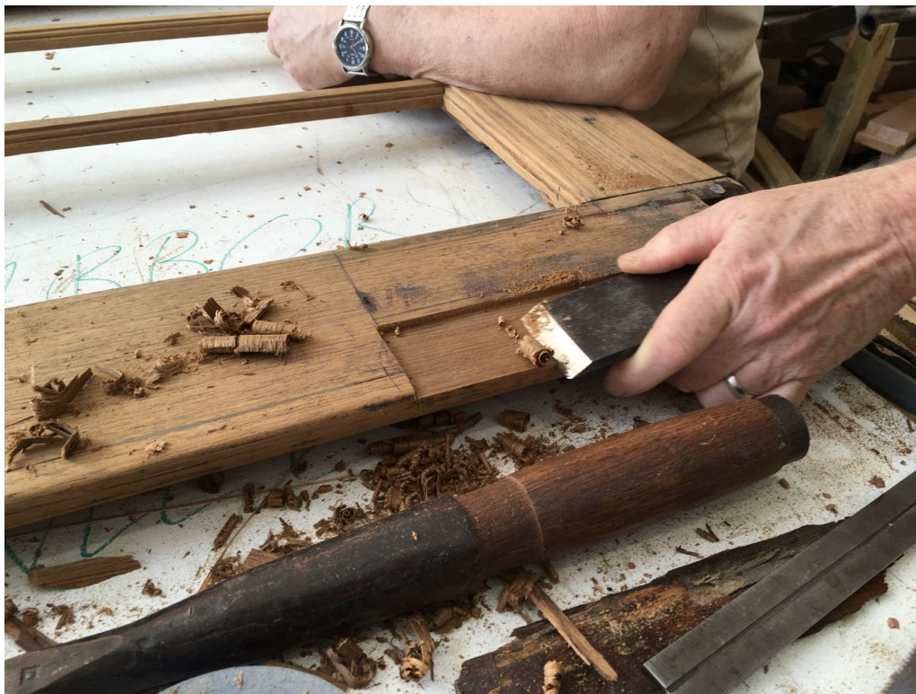
Figure 29: Lou at work with a large 'slick' chisel
