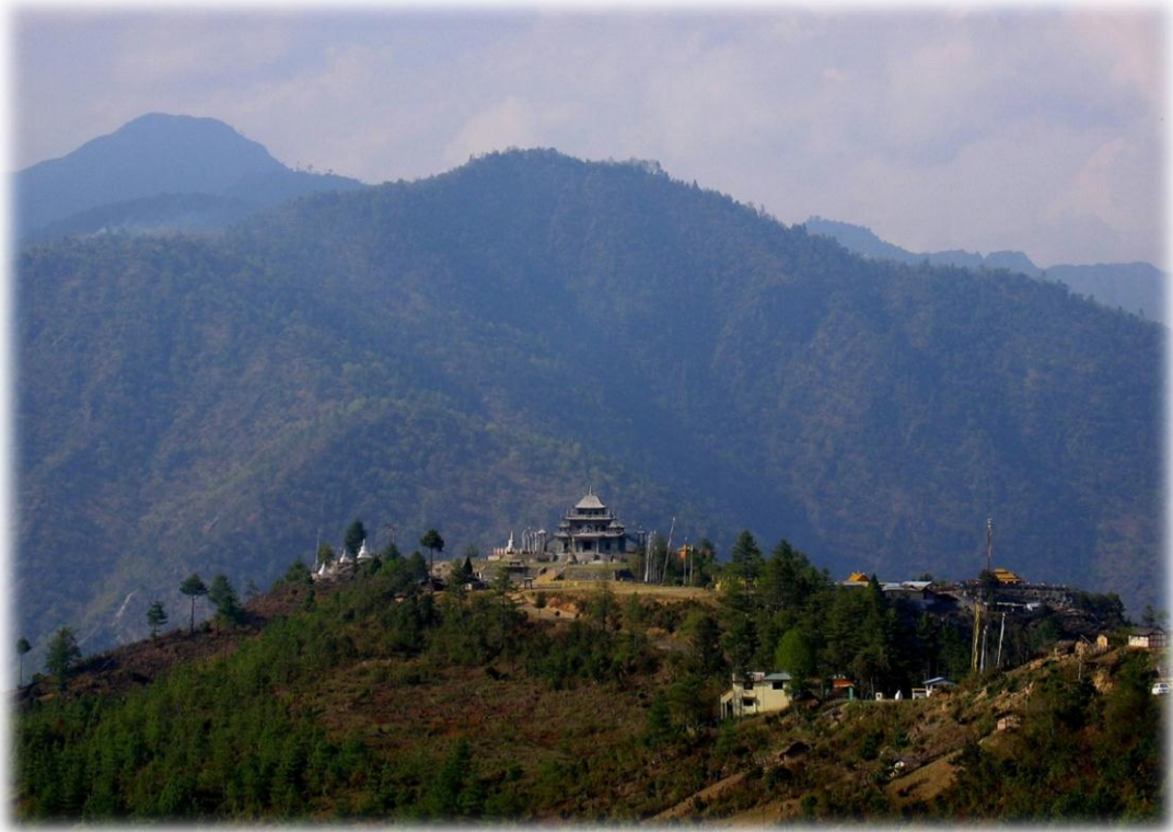
Figure 25. Zangdokpalri temple under construction in 2006.
