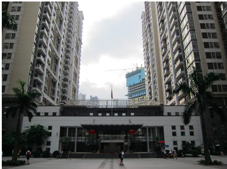
Figure 8.2. The new office building of Liede Economic Development Company. Source: Taken by author September 24, 2013.
