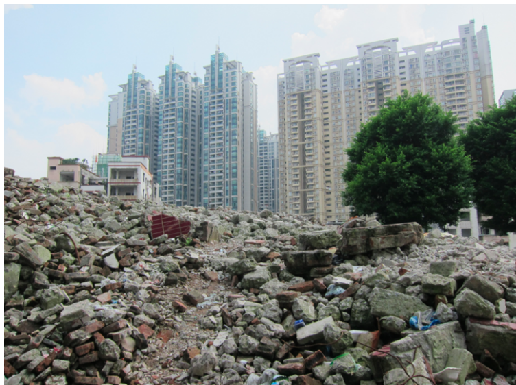
Figure 8.5. Xiancun during demolition. New residential developments lie just blocks away from the ruins. Source: Taken by author September 25, 2013.
