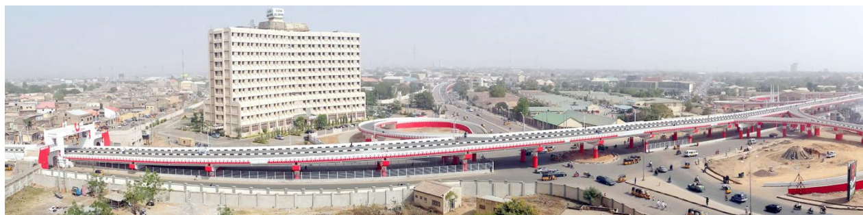
Figure 7.23: Flyover constructed by the Kwankwaso government painted in the red 'Kwankwasiyya' colour
