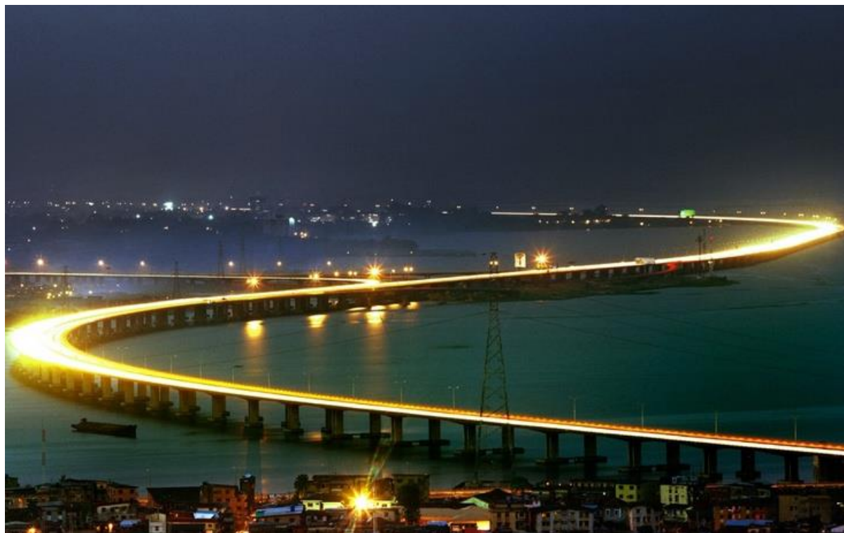
Figure 6.11: The Third Mainland Bridge, linking the Lagos Island to the Mainland
