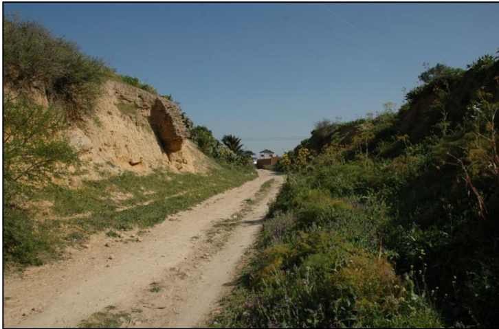
Fig. 14: Masonry substructure of the aqueduct crossing the ravine between the amphitheatre and the 'citadel'.
