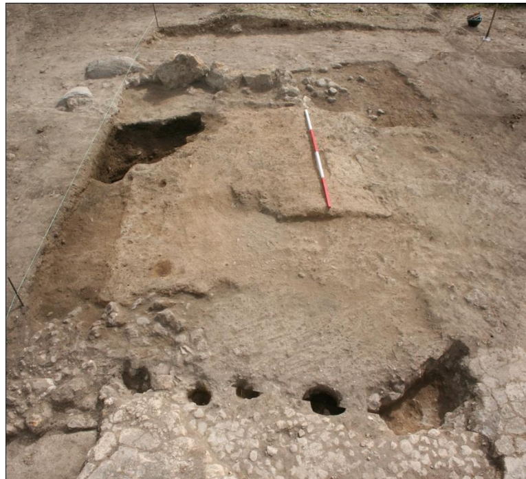
Fig. 24: Building 3, its structure defined by postholes and robber trenches. From the north.
