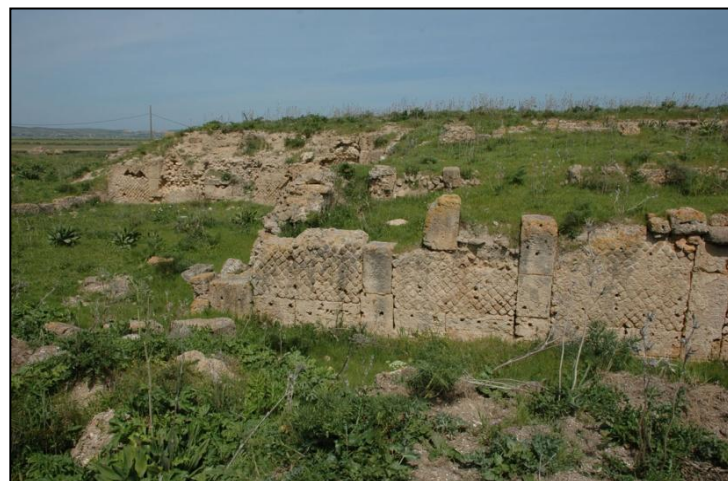
Fig.19: Structure in a mixture of opus reticulatum and opus africanum , with clamp holes for marble veneer panels.
