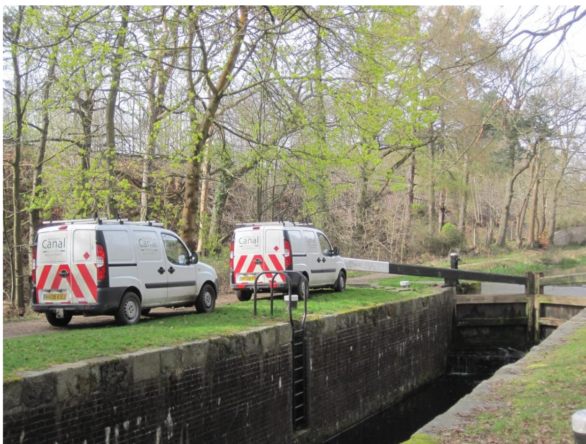
Figure 3 Two vans belonging to the Basingstoke Canal Authority, adjacent to the canal at Deepcut Locks
