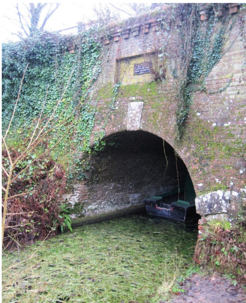
Figure 24 Greywell Tunnel, eastern portal
