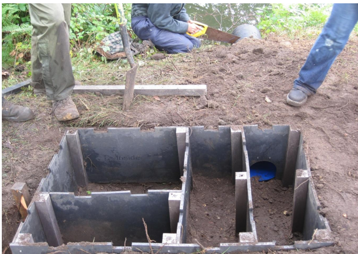
Figure 32 Installation of otter holt
