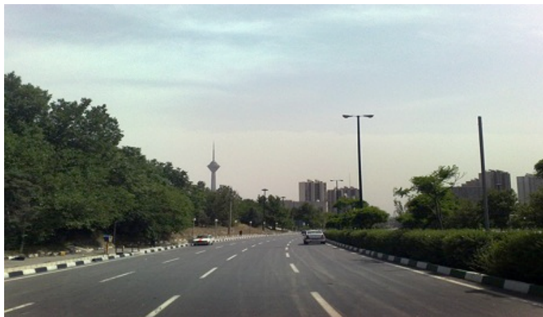
Figure 8.4: Milad tower and freeway in Shahrak-e-Garb, North of Tehran that is yet to open and be fully functional’, LGOIT June 2010 archive (07/06/10).
