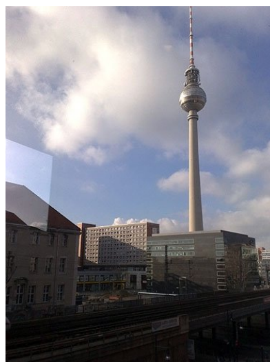
Figure 8.5: ‘The Fernsehturm (Television tower) in Berlin, located near Alexanderplatz’. LGOIT 2008 archive (21/12/08).
