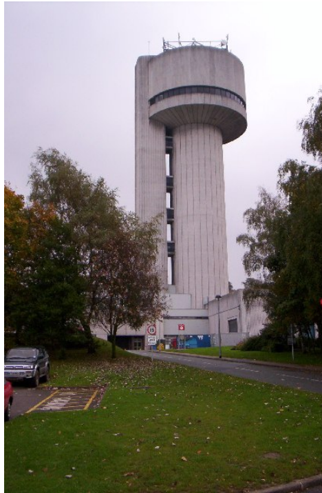
Fig. 1.2: The building of the large laddertron charged electrostatic accelerator at Daresbury. The terminal with the ion source was at the top and the accelerating column went down the whole tower towards the bottom. The accelerator was shut down in the 1990's. Picture taken from Wikipedia (user: Jotelcommons) under the creative commons licence CC BY-SA 2.0
