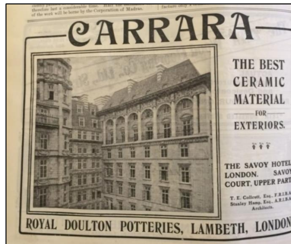
Figure 14 'The Best Ceramic Material for Exteriors'. Doulton's Carrara at the Savoy (1909) 301
