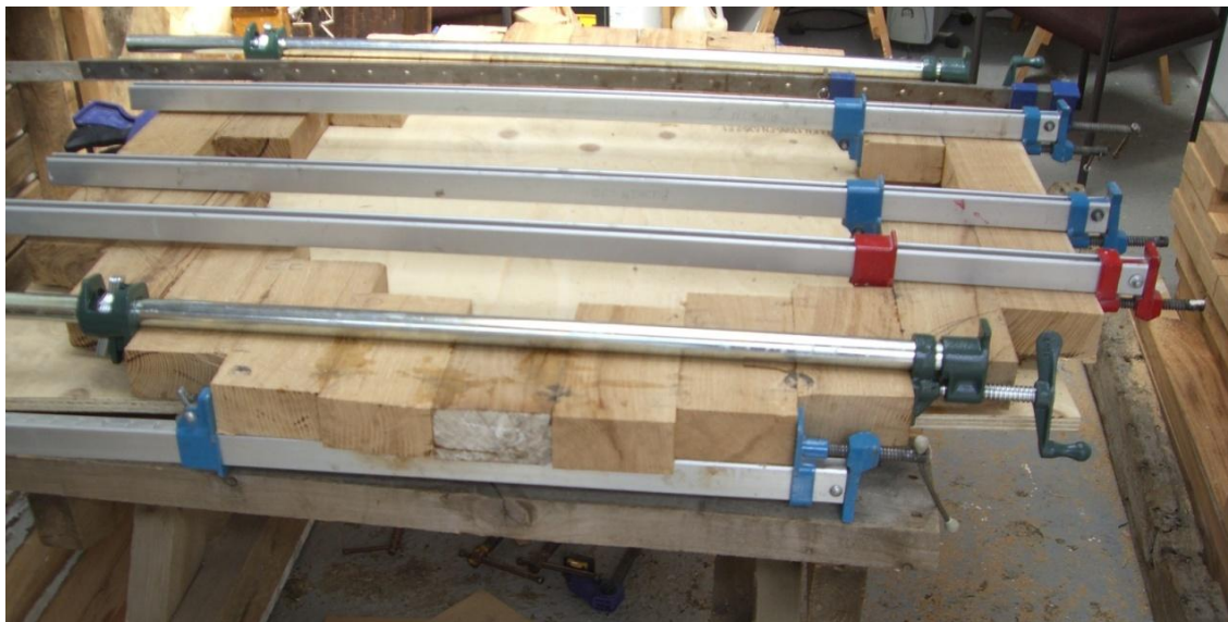
Section of the sphere being glued together
